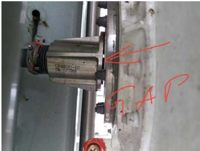
Loose main landing gear door fitting – notice gap
